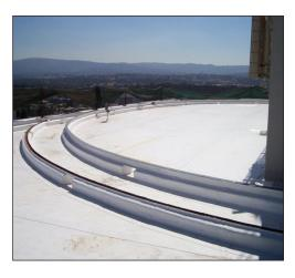
On a hot day, the white membrane will measure only 91° F compared to a black roof that reaches 172° F. This is possible because the IB roof membrane can reflect up to 90 percent of the heat from the sun which would otherwise enter the building. Additional savings to the building manager can be achieved as new air conditioning units are downsized because of a reduction in load on the HVAC system.
