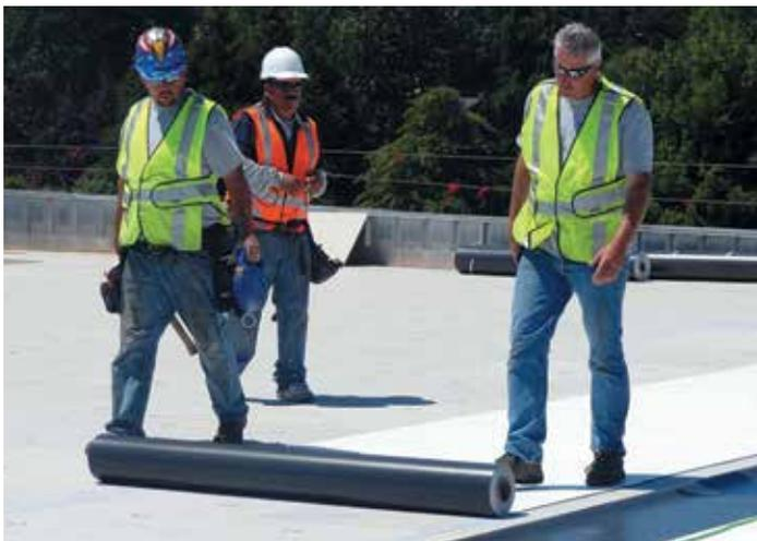
**Figure 4. Worker laying out roof roll.**
