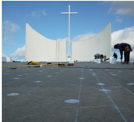
After removing the copper roof, Sharpe Inc. added a second layer of 2-inch ISO insulation over the existing plywood. Next they installed 3-inch plates using heavy-duty screws to fasten the insulation. Sharpe Inc. used the FM I-90 pattern for uplift, one fastener per 2 square feet over the entire roof.
